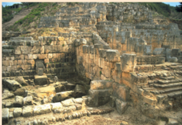
View showing various levels of construction
